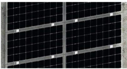
The horizontal and vertical distance between the modules is 10 mm.
